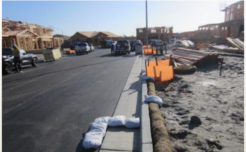
Gravel bag check dams in curb flow lines
