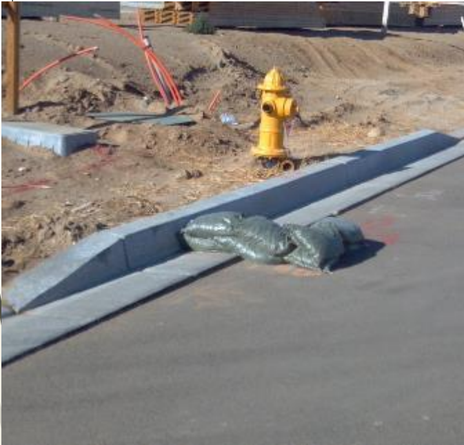
Gravel bag check dams in curb flow lines
