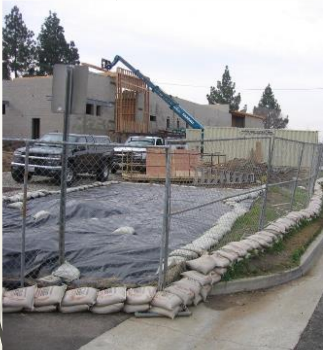
Multi-layer gravel bag linear barrier.
