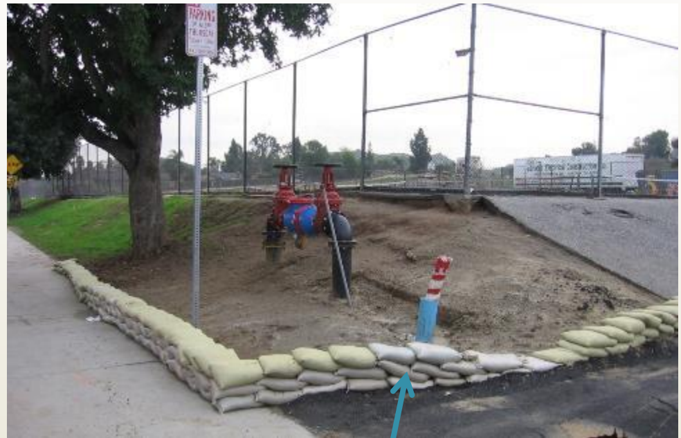
The ends of the bags should overlap.
